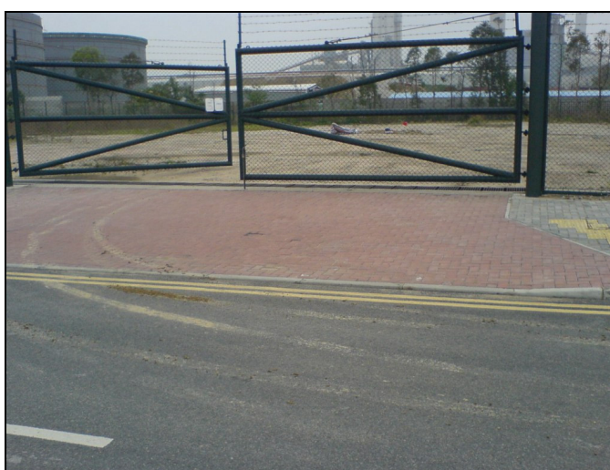
Photograph 8-1 Soil Debris on the Road Outside EP08-01
